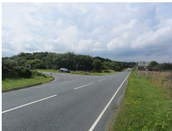
Photograph 14. A171/Egton Low Moor junction for access to Lady Cross Plantation. Load approaches camera and turns right.
