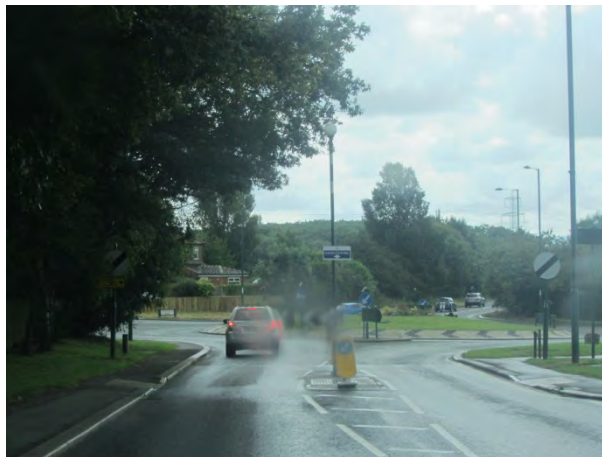
Photograph 3. A171/A1043 roundabout. Load moves away from camera and turns left. Low level kerb and removeable street furniture enable use of full road width.
