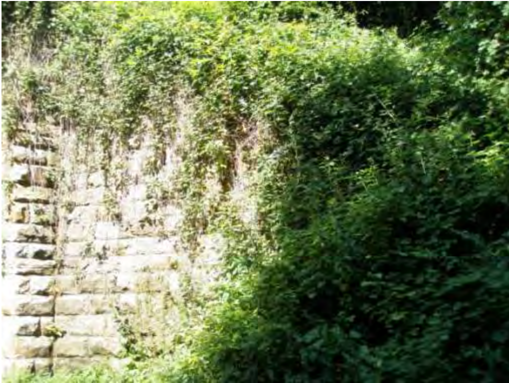
Photograph 5 (P3) - South east wing wall
