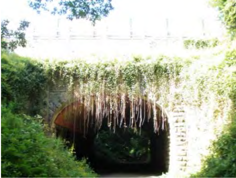
Photograph 1 (P1) – South elevation
