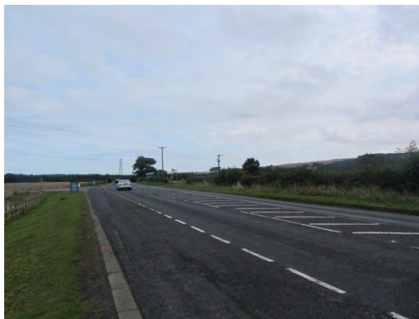
Photograph 6. Tocketts Mill site access looking east. Load moves away from camera. New access road to be constructed on the right.
