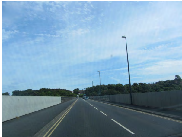
Photograph 24. A171 Whitby New Bridge at OS Reference NZ 101 899 over the River Esk looking south.
