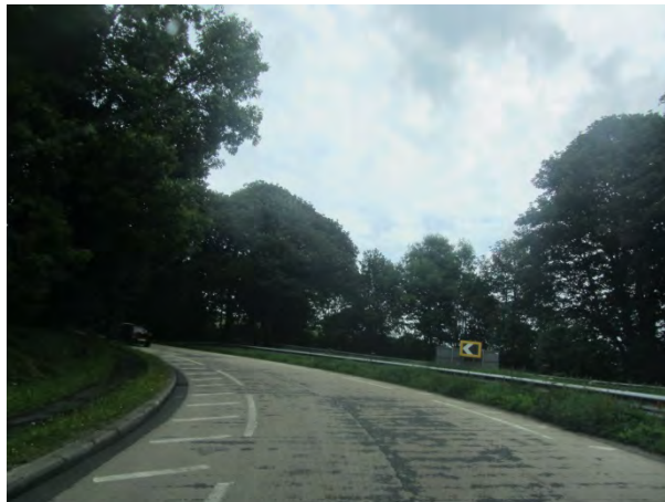
Photograph 8. A171 approach to Aysdale Gate. Load moves away from camera on a steep gradient. Wynns considers this incline accessible for the proposed transport arrangements. In the event that weather conditions were poor then additional tractor units could be utilised to assist. Load would be taking up full width of carriageway at slow speed.
