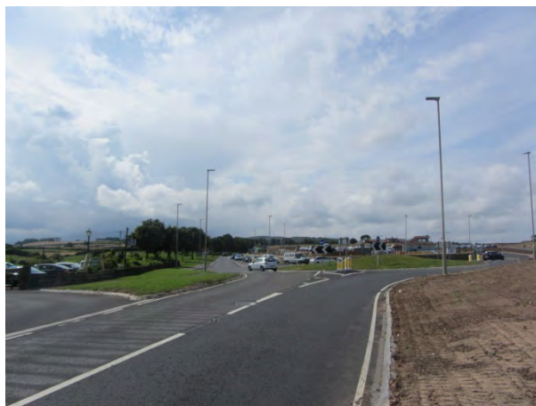
Photograph 17. New Roundabout on A171 at north entry to Whitby adjacent to new Park and Ride facility. Load approaches camera. Possible contra flow suggested.
