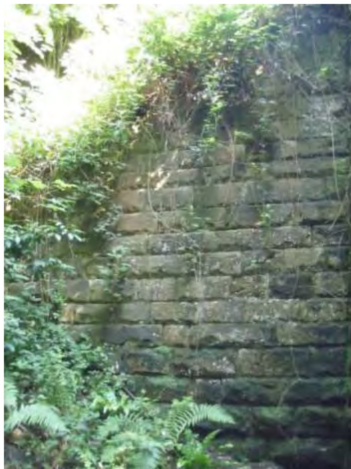
Photograph 8 (P22) - North east wing wall
