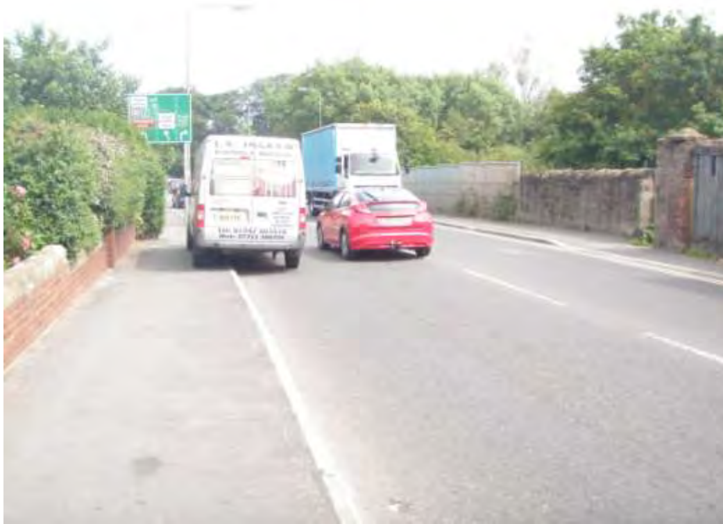
Photograph 3 (P26) - West approach
