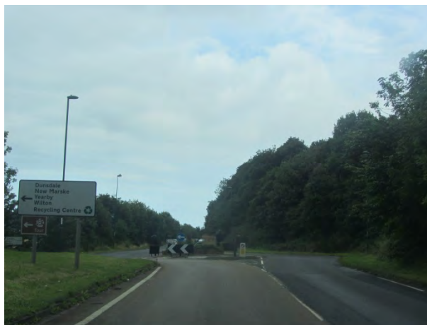
Photograph 5. A173/B1269 Tocketts Mill straight on. Caution camber to be noted by haulier. Could be contraflowed if required to avoid camber.
