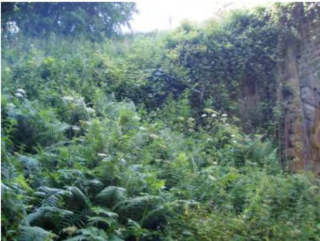
Photograph 6 (P4) - South west wing wall
