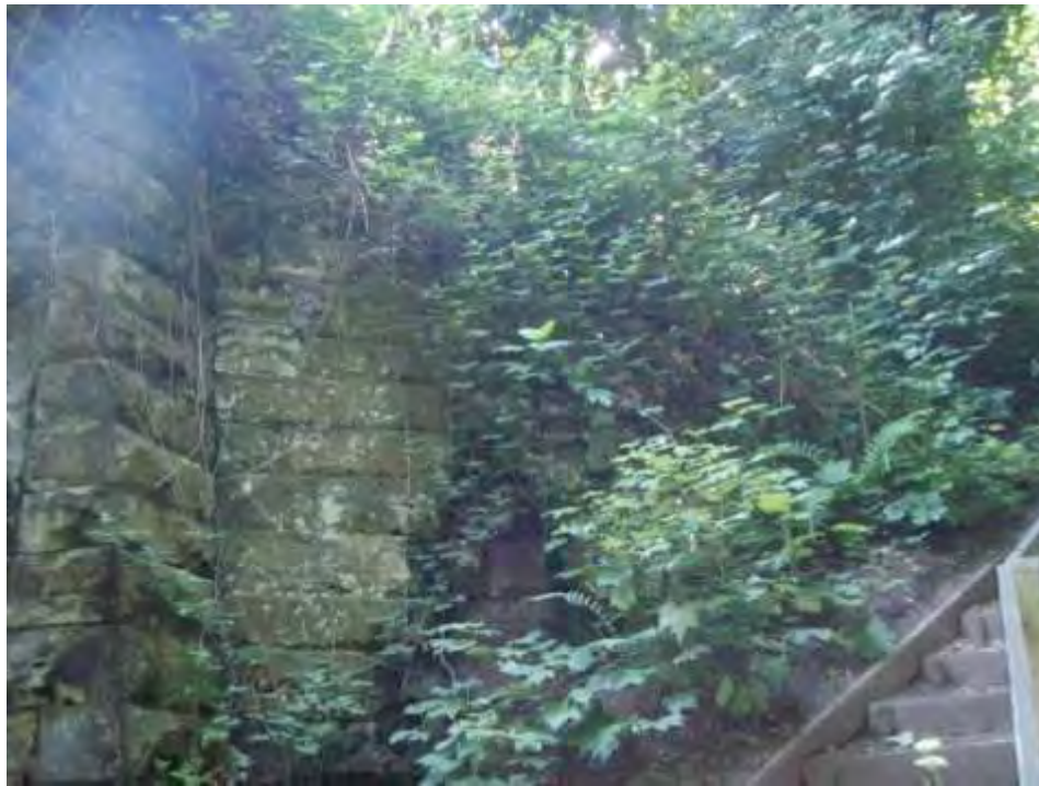
Photograph 7 (P21) - North west wing wall
