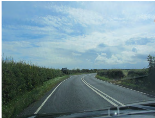
Photograph 26. The series of bends known as Normanby Bends are all negotiable for the proposed loads. Load moves away from camera.
